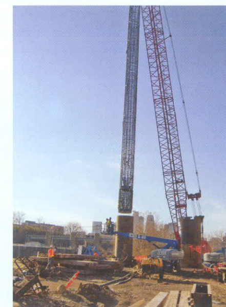
Osterberg Cells being placed
