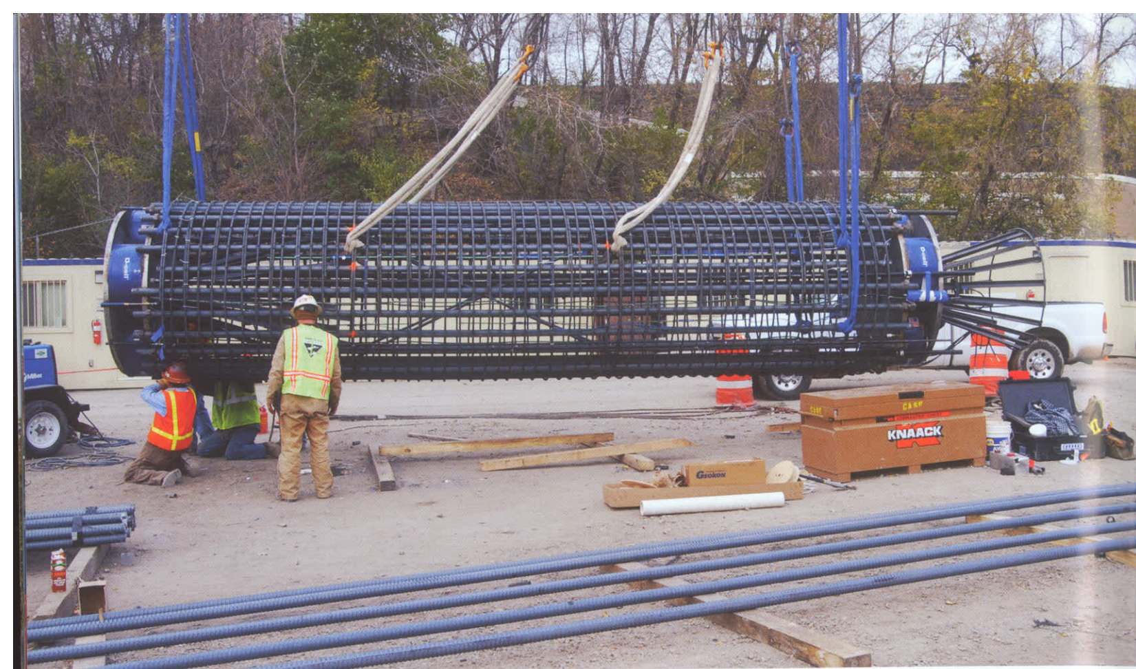
Level Osterberg Cell on site for Minneapolis's I-35W replacement bridge
